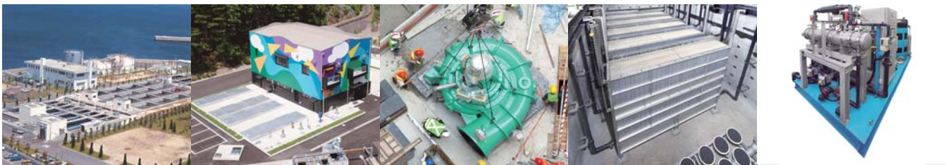
Sewage Treatment Plant
