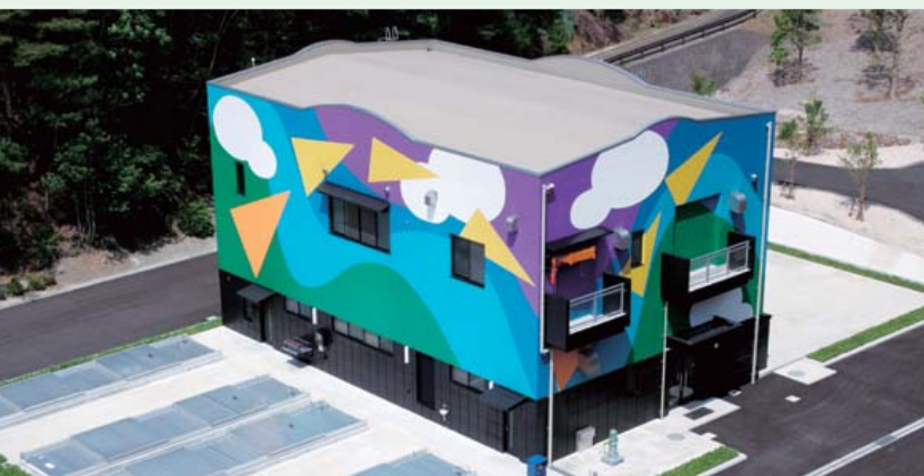
Water Purification Plant
