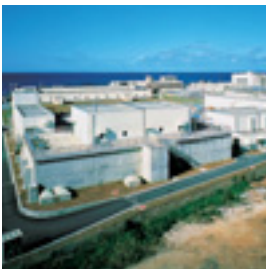
Advanced Water Treatment Plant
