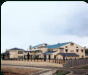
NIGHT-SOIL TREATMENT PLANT
