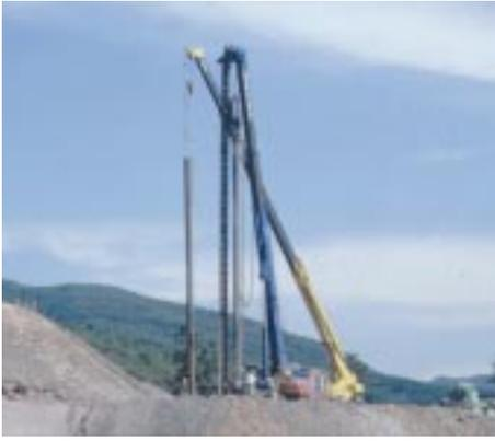
*G-piles, cast steel pile for civil engineering*
