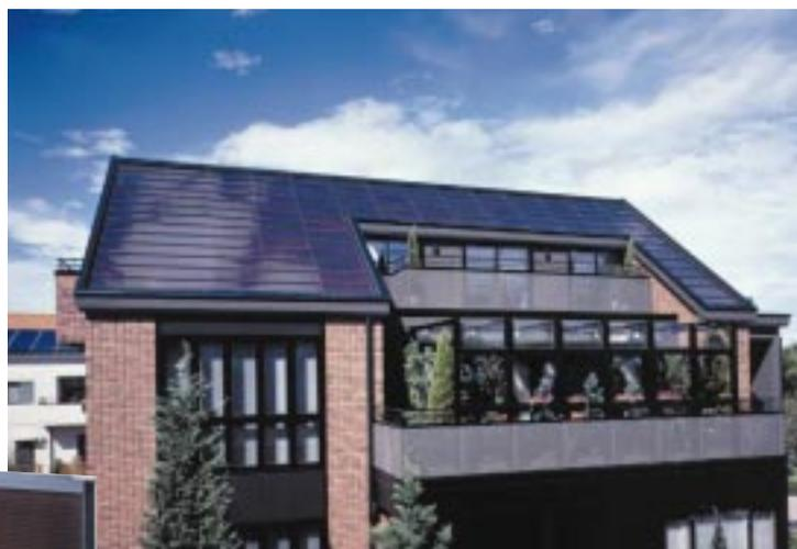
Roof-system fixed photovoltaic (PV) shingles: Model "Ecolony"
