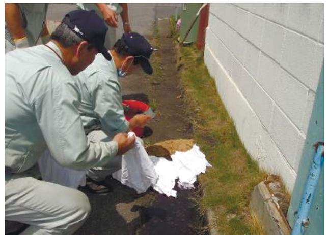
Absorbents were placed around the spill to prevent its further spread.
