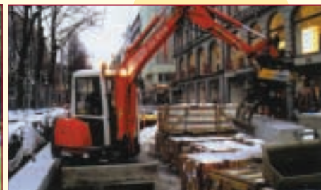
Mini-excavator with new-type engine at a construction site
