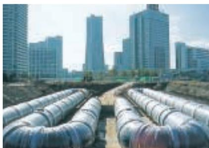
Water storage tanks using ductile iron pipes
