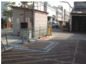
The measure for leak of heavy oil at intake from tank truck (Sakai plant) (installation of ditch for collecting oil)
