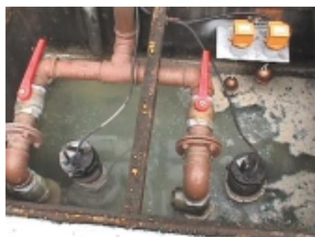
The prevention of wastewater over flow at an accident by dual pumps (one of them is a spare pump in an emergency) (Sakai plant)
