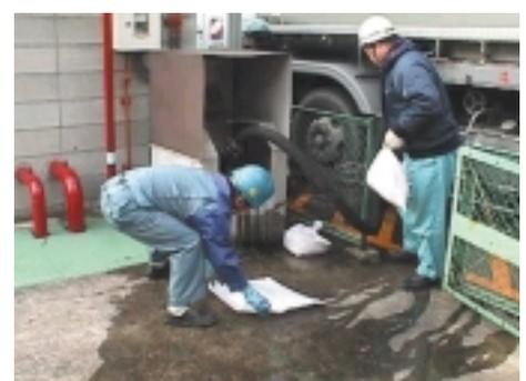
The training view of heavy oil leakage from the flange connection at intake from tank truck (Sakai plant)
