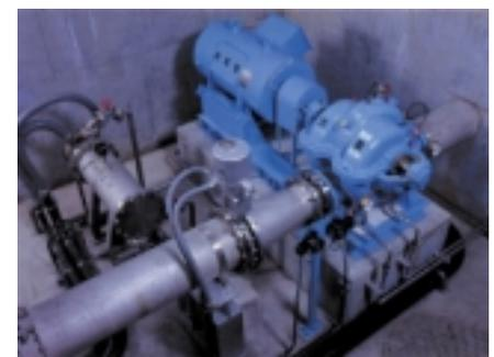
Pump with reverse rotation impeller
