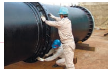
KUBOTA's new joints were adopted by the U.A.E. for their 47-km pipeline composed of huge 1,600-mm-diameter iron pipes.
